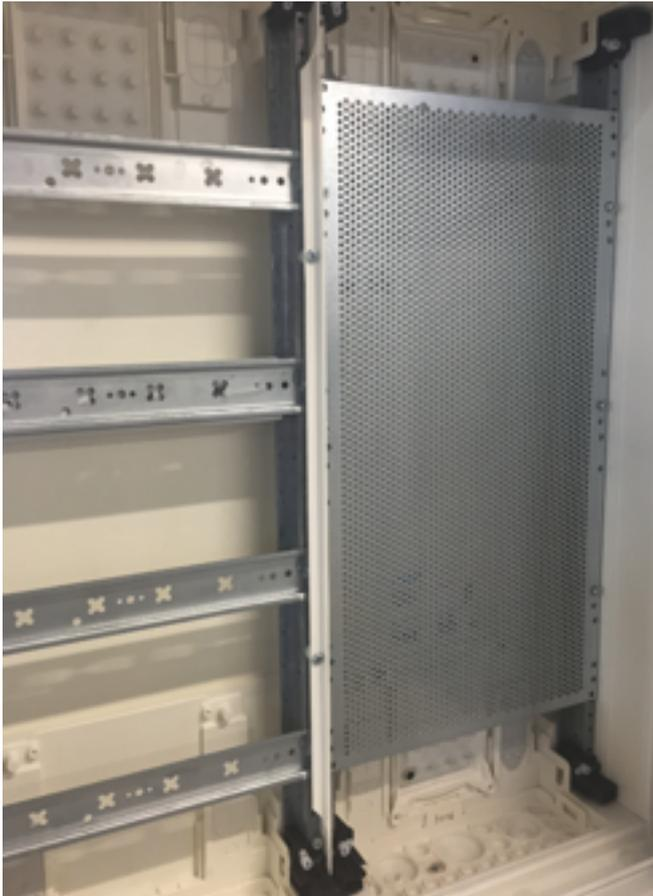
Installation of UZ40F1 in FWB distribution board, size 42:
